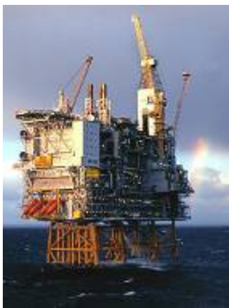
Fig. 1a. Grane offshore platform, operated by StatoilHydro in the Norwegian Sea off the coast of Bergen, Norway.
